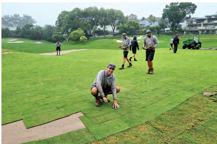
Pictured top: Slotted drainage pipes were installed in the green bases so that the club could, if it chose to in the future, purchase SubAir units and connect them; Middle row: Major changes were made to the par three 11th with construction of a stone wall and creek system (left), while the greens sand was amended with coir fibre (right); Above: Greens were solid turfed so they could be brought back into play quicker
