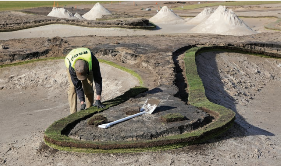
A unique combination of synthetic and natural sod revets is being used to construct the new Royal Sydney bunkers
