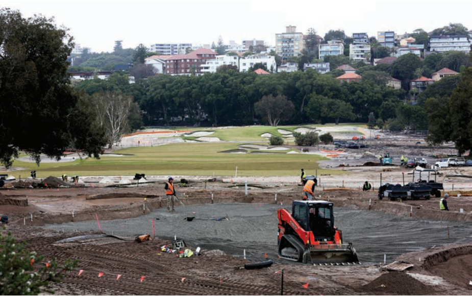
The new Royal Sydney greens feature a perched water table construction along with Sub Air infrastructure
