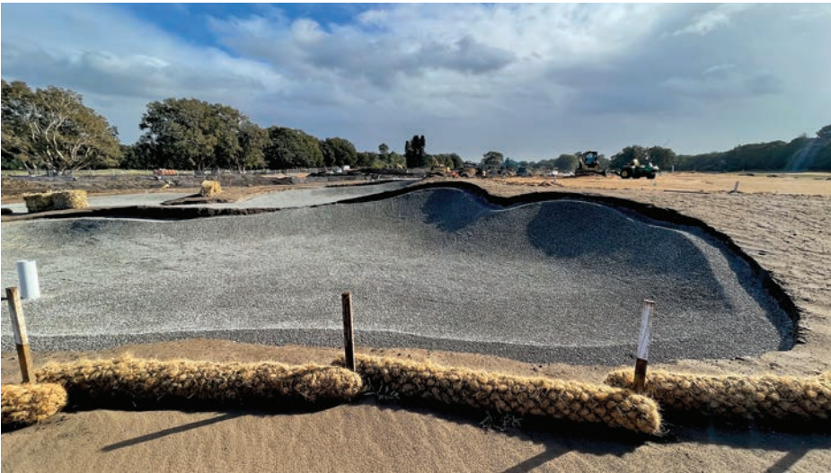
Royal Sydney is using the Better Billy Bunker Method in its bunkers which comprises a locally-sourced gravel spread to a 50mm depth and then sprayed with a binding polymer. The photo shows how the gravel goes up and over the 300mm hand-excavated ‘bench’
